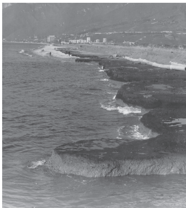
Fig. Erosion profile near Gagra showing upper Holocene marine deposits overlying a middle Holocene peat formation (PhotoV. Peshkov).
